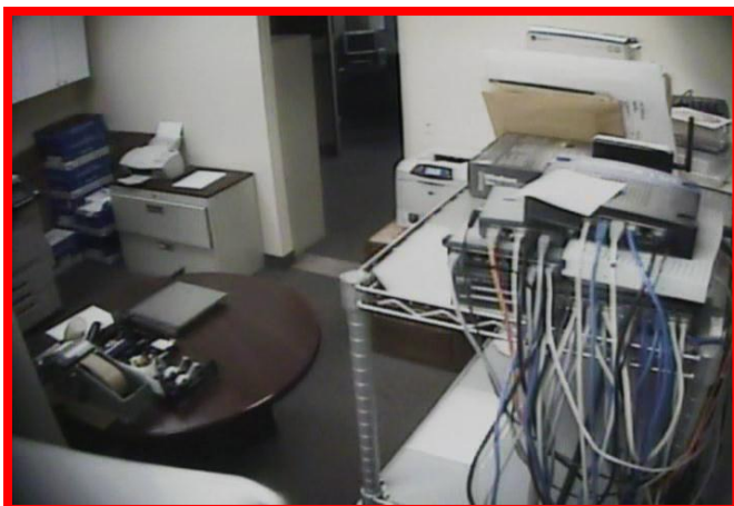
Figure 14. INEFFECTIVE – Multiple obstructions blocking the camera view.
