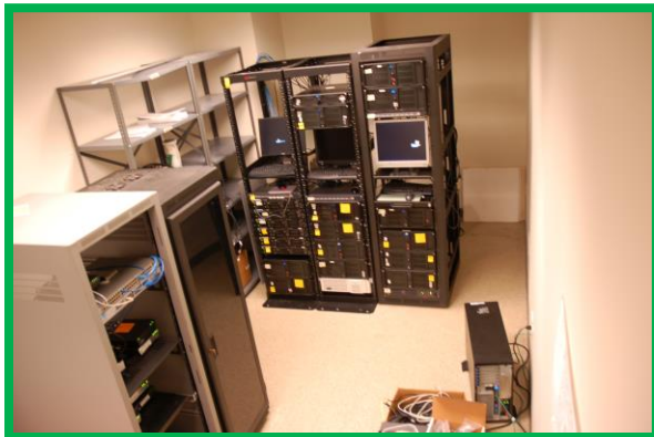
Figure 24. EFFECTIVE –The camera view includes as wide a view as possible. A person standing in front of the area of most interest (in this case, an equipment rack housing computers), would be in full view.
